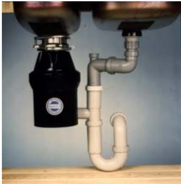
Figure 6. Kitchen waste disposal unit mounted under a sink
